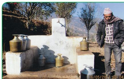
Water supply in Makawanpur
