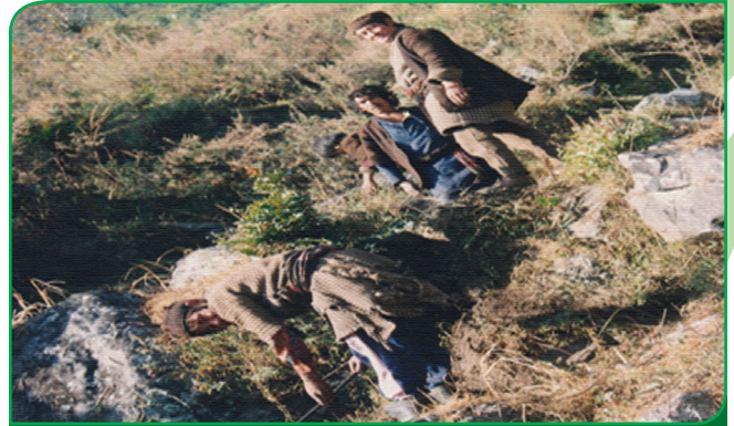
Figure 2 Digging water pipeline in Grey, Rasuwa -1993
